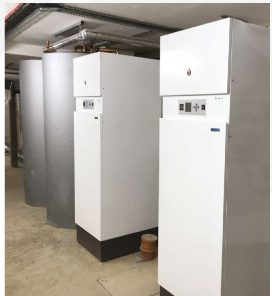
HR cylinders (grey) and HeatMaster® combi boilers provide hot water to the student accommodation.
