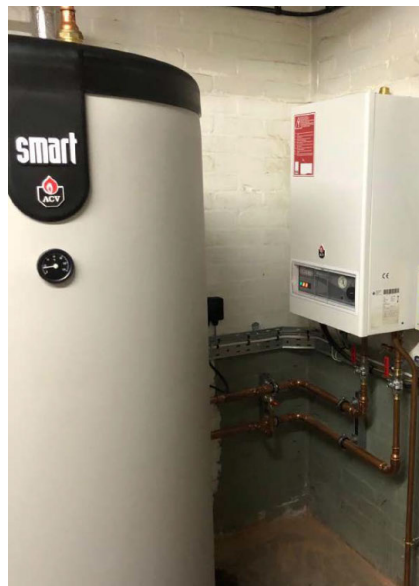
The ACV electric boiler and Smart tank combination provide a compact and efficient solution with no gas required.
