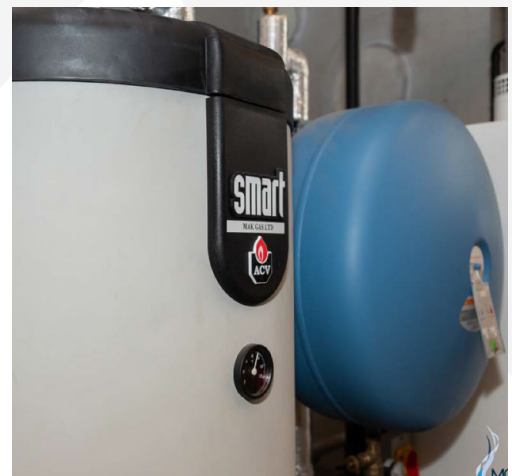
The Smart tank-in-tank cylinder provides quick recovery domestic hot water to meet the needs of the schools' bathrooms
